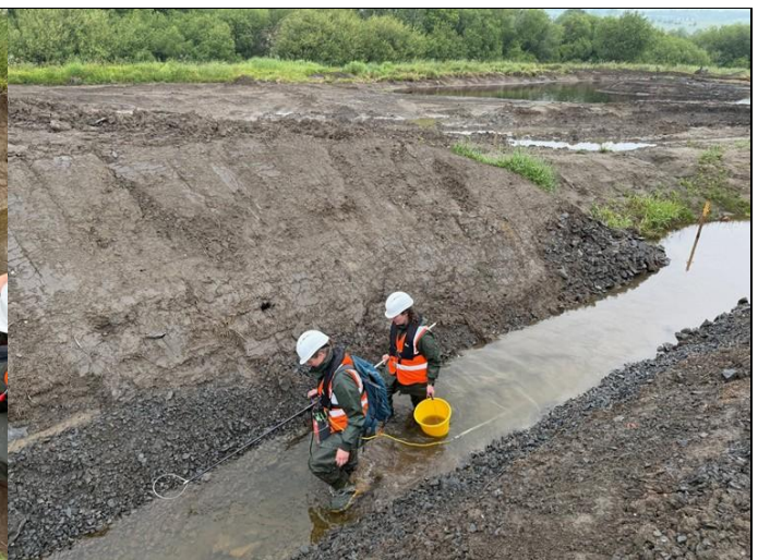
Fish rescue in site of culvert installation
