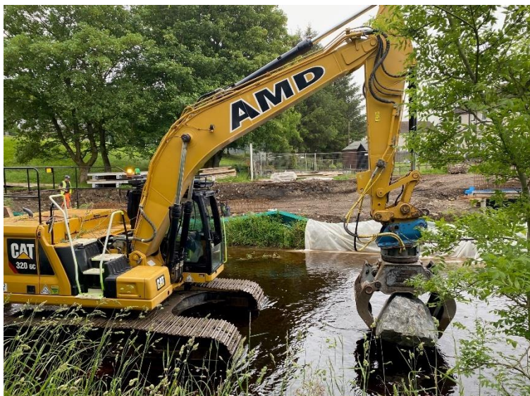
Stone placement in the Afton Water
