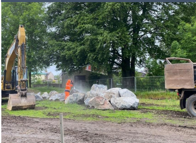
Stone cleaning prior to entering the Afton Water
