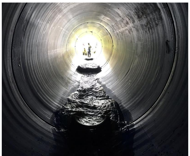
Baffles installed inside the culvert
