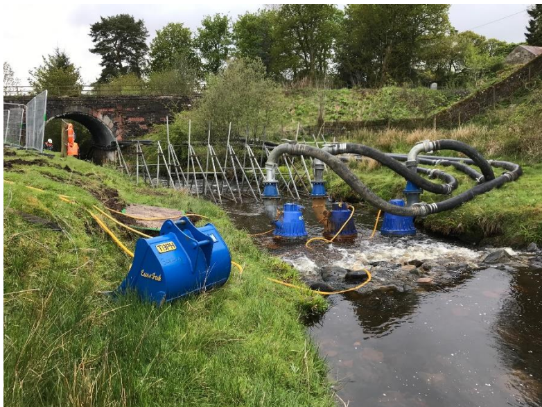
The Polbower Burn being over-pumped to allow engineering works
