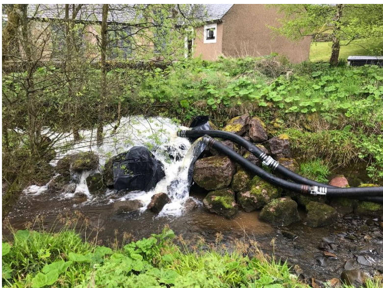
Water outflow being safely discharged onto the riverbank to prevent scouring.
