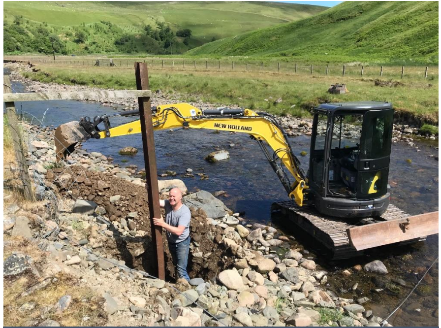
Metal posts being installed for the watergate by C & K Harvey
