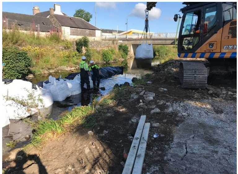
Sandbags being placed in-river prior to works commencing
