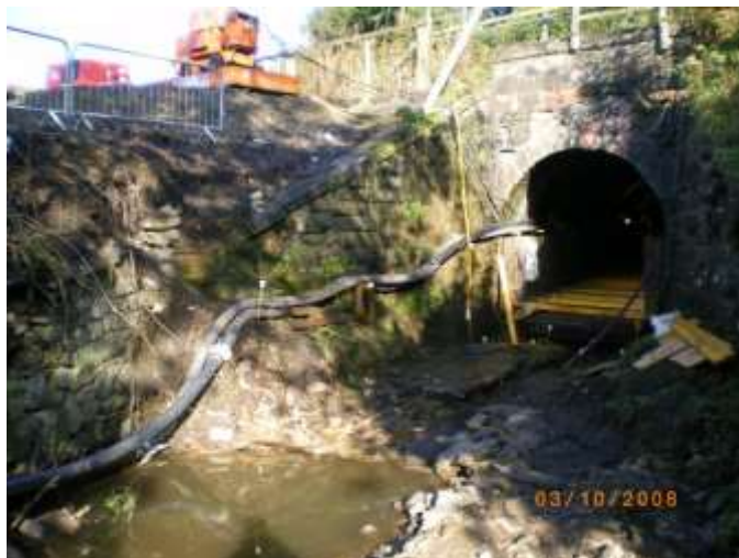
Engineering works at Hallburn
