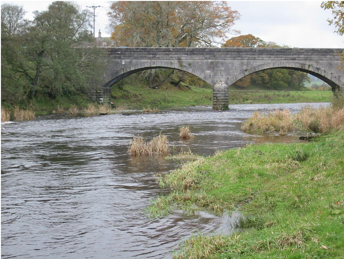
River Nith, Blackaddie Bridge, Sanquhar.
